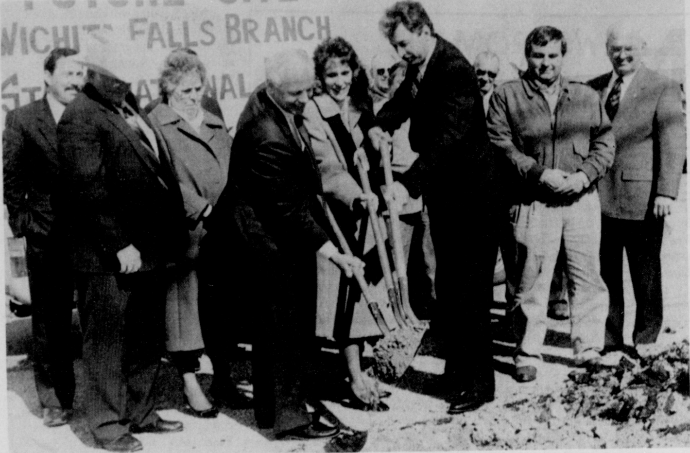
IT'S OFFICIAL - A ceremonial ground-breaking, signaling the start of construction of the Wichita Falls Branch of State National Bank, was held Tuesday afternoon at the Thaten Shopping Center on Old Iowa Park Road. Operating the shovel are, from left, Gene Jordan, SNB president, Michelle Wells, who will be assistant manager, and Bill Hoffman, manager. Representatives of the SNB and the bank's parent company, North Texas BankShares, attended, including Stanley Williamson, president, on left with hat.
