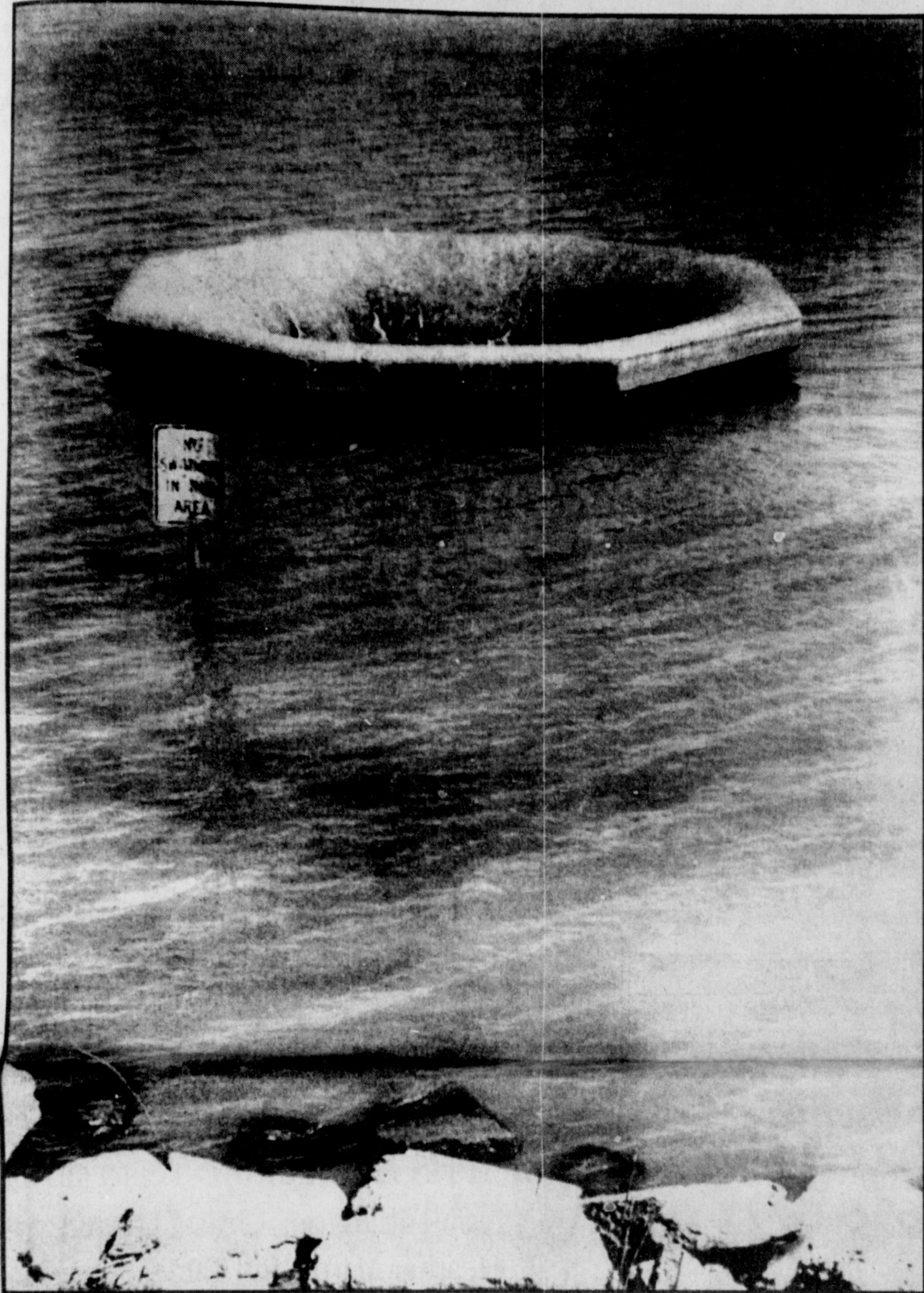
RECENT RAINS, such as the three-quarters of an inch Iowa Park received over the past weekend, have benefited Iowa Park's two water-supply lakes. This was the scene at Lake Iowa Park Tuesday, when the water was a foot and a half below the overflow flume. That lake is slightly more than a foot below its level this time last year, but has risen some three feet since April 3. Lake Buffalo is less than seven feet below its overflow, but has held its own since November, according to measurements taken by city workers.
