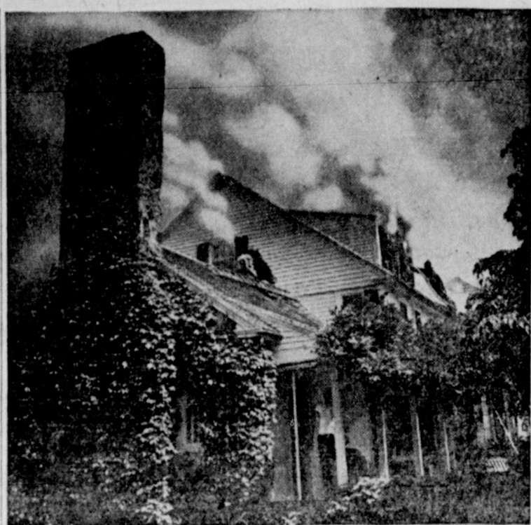
Sparks from an incinerator ignited the flammable roofing on this historic home in Bloomfield, Conn. Only quick action by firemen prevented flames from destroying the $50,000, pre-Revolution structure, a gun mill in the early 18th century.
