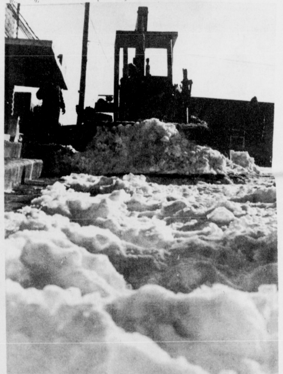
PILING UP THE DRIFTS ...city crews clear streets of snow.
