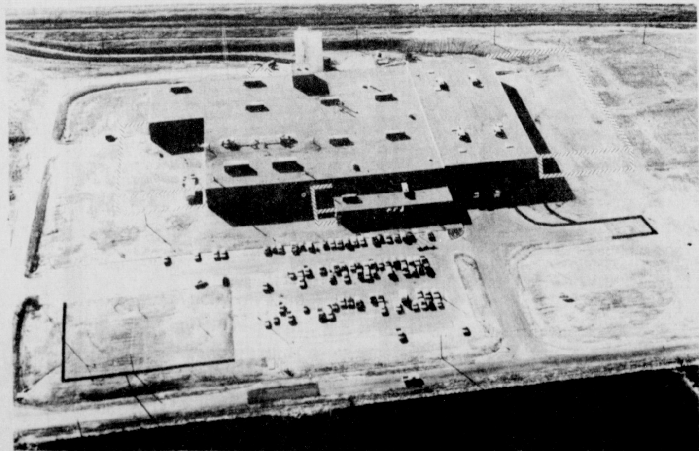
CRYOVAC EXPANSION areas are outlined by lines on all four sides, plus darkened parking area expansion in this aerial view of the plant site on West Magnolia. At left is new manufacturing space; at right is new warehouse space. The small addition in the front is for expanded canteen and office space. At the rear, to the left of the silos, is a new ink room. Black lines in front indicate expanded parking and driveway pavement.
