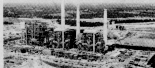
Two lignite coal-fired units are already generating electricity at the Monticello plant near Mt. Pleasant. A third unit is also under construction there.
