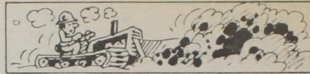
More than 1.2 million cubic yards of earth and rock had to be excavated from the site of Manhattan's World Trade Center before building could commence.
