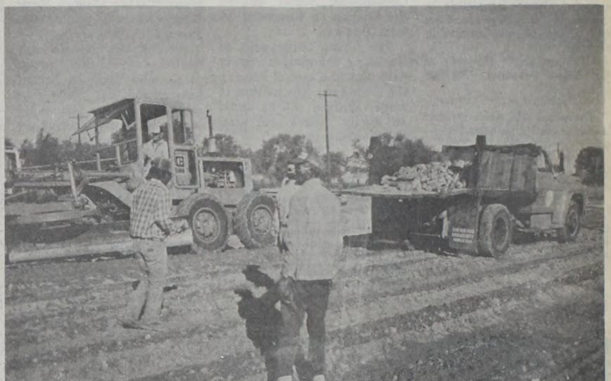
Turkey City employees preparing road bed for new street paving.
