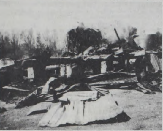
THE FORMER TEXACO WAREHOUSE EAST OF THE ELEVATOR IN TURKEY.
