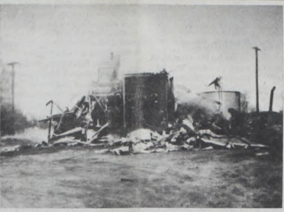
REMAINS OF THE TURKEY ELEVATOR AFTER SATURDAY NIGHT'S FIRE.
