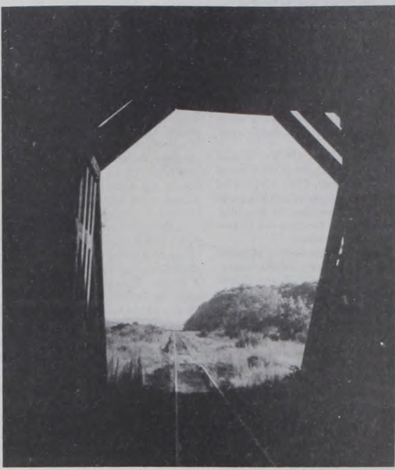
Looking southward into the canyons through the tunnel, this photo by Trent McKay, contrasts the darkness of the tunnel with the beautiful scenery outside.
