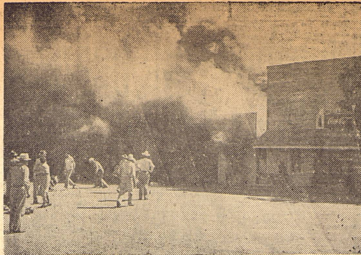
business block as work continues in the removal of merchandise from Willett's Grocery of the two-story Masonic building and the adjoining small structure used for storage by Killion's Red & White Grocery. The Masonic Lodge of May occupied the second floor of the building at right. The community public scales and the small structure with them, back of the above buildings, also were destroyed.—Photos courtesy Brownwood Bulletin.
