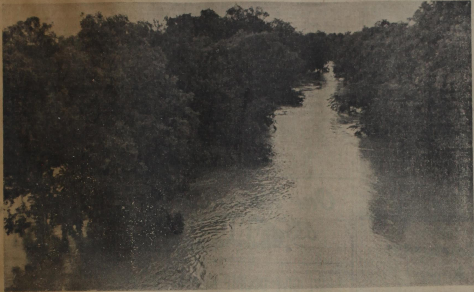
BAYOU ON RAMPAGE — Pecan Bayou, where it crosses State Highway 279 just south of the Cross Cut com-
