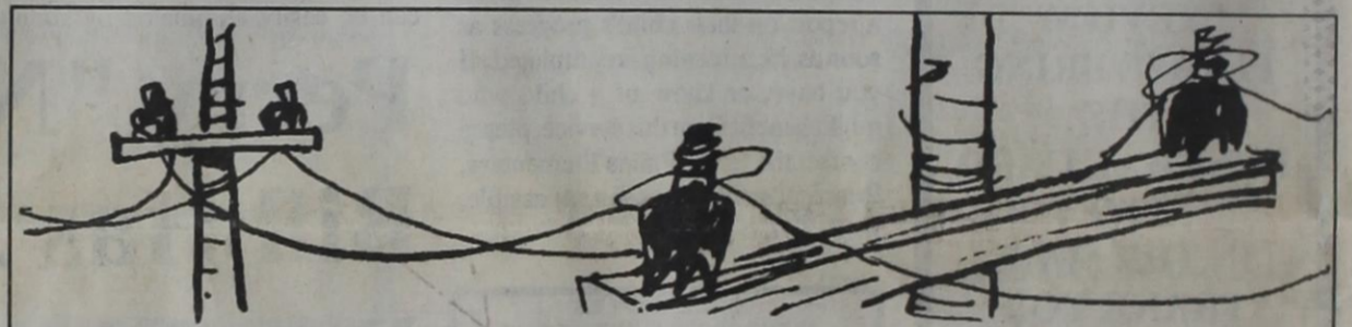
When the first long-distance telegraph cable was laid in 1844, it was strung on wooden poles and the necks of broken bottles for insulation.
