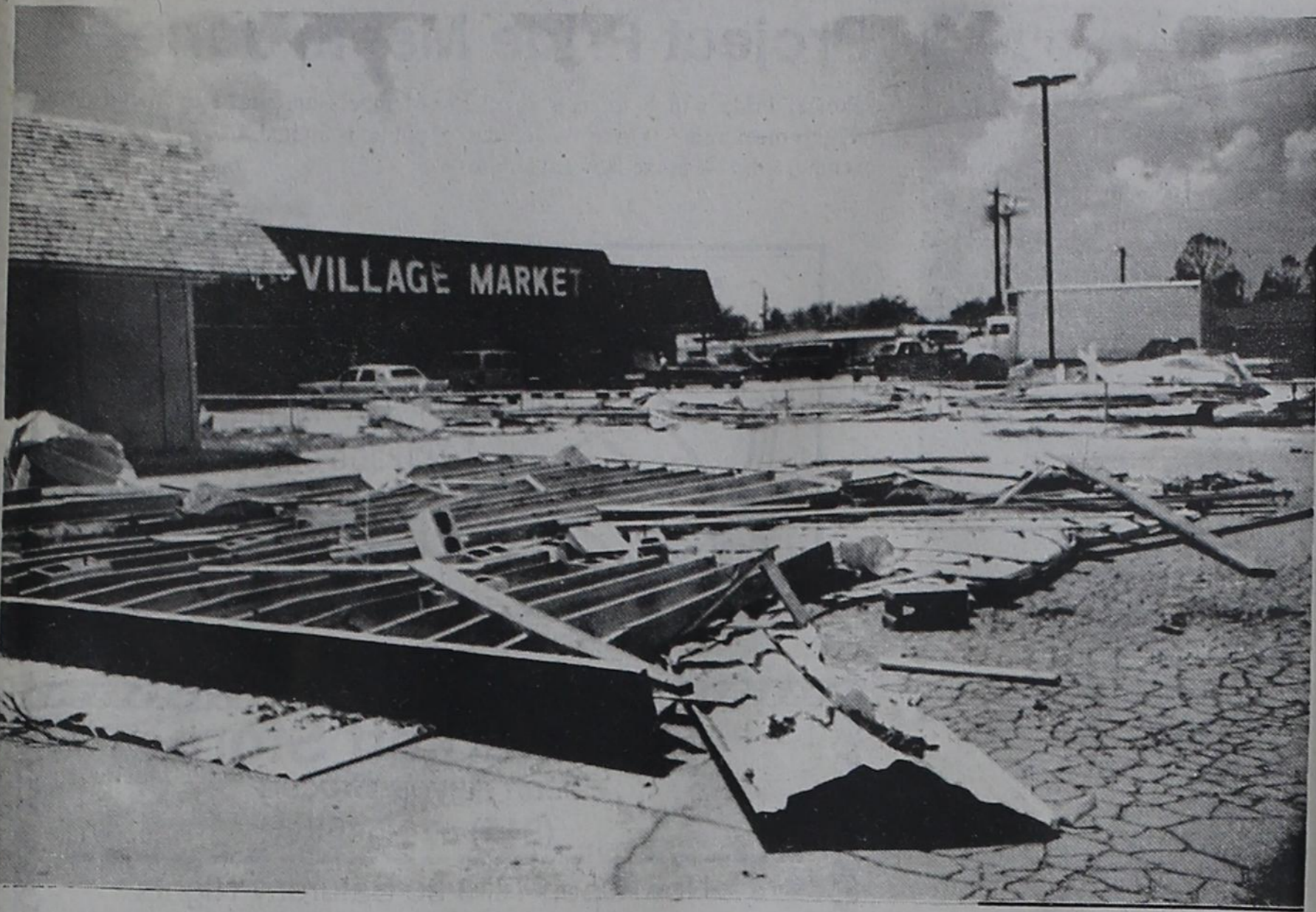
JACK'S PLACE ROOF IN BONNIE'S STAINED GLASS PARKING LOT
