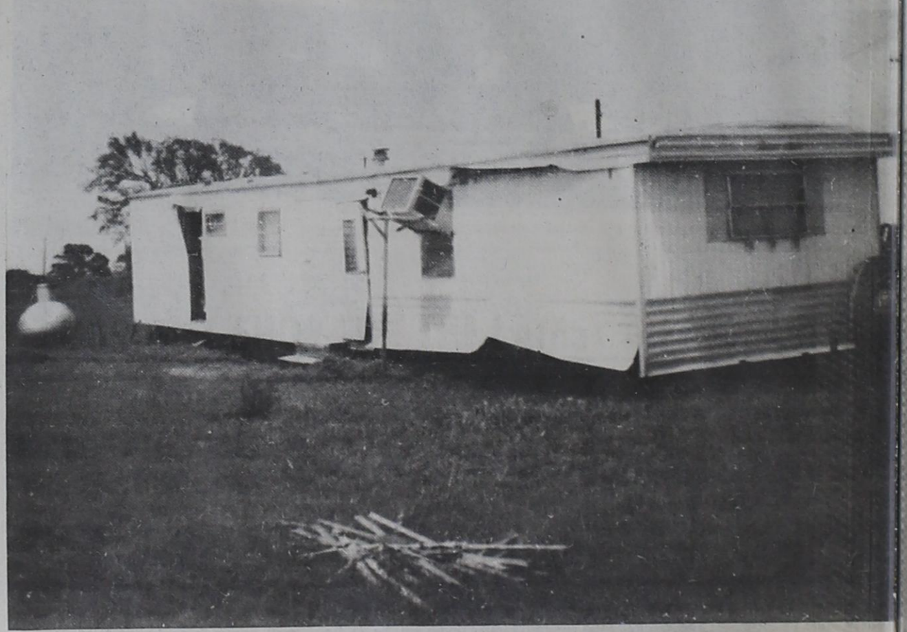
MR. AND MRS. ROBERT PICKETT'S MOBILE HOME DAMAGED AT CROSS CUT
