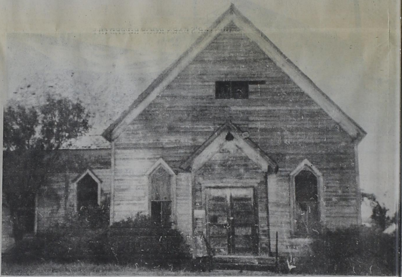
CROSS CUT CHURCH MOVED OVER ABOUT 1 FOOT FROM ORIGINAL STEPS
