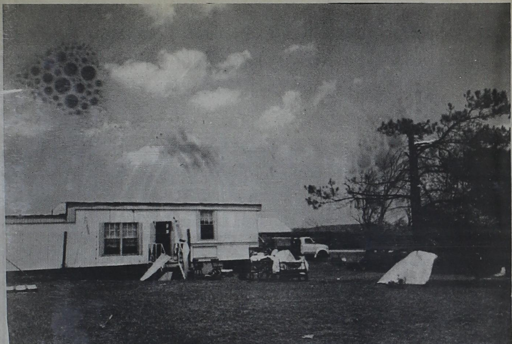
MOBILE HOME AT COTTONWOOD DAMAGED SEVERELY
