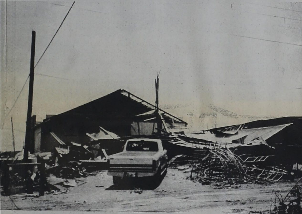
LAWRENCE FARM & RANCH SUPPLY, INC. WAREHOUSE DESTROYED
