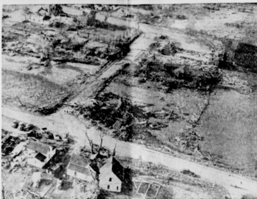
HAVOC IN WAKE OF TWISTER . . . Here's an airview of the extensive damage wrought by tornado which swept through Duncan, Iowa, population 100, recently. There wasn't a house left undamaged by the freak twister which caused one million dollars damage and injury to five persons.
