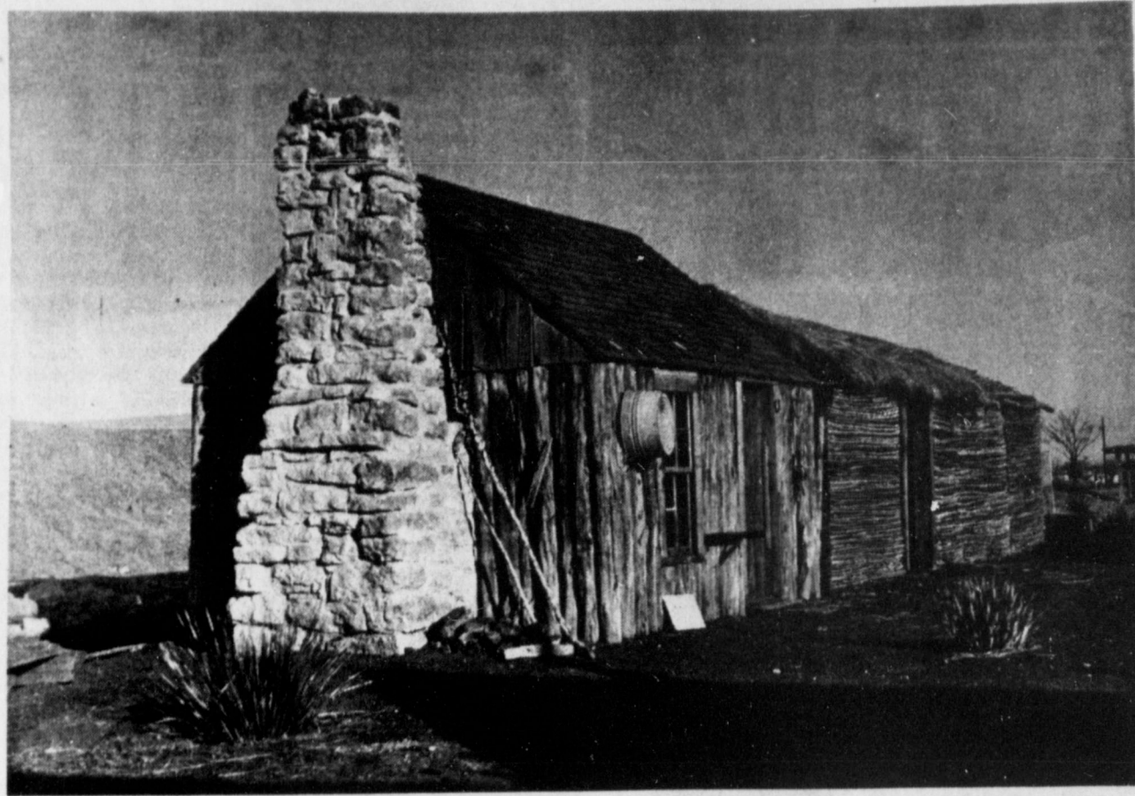
PICKET AND SOTOL HOUSE — The Ranch Headquarters Association recently dedicated this Picket and Sotol House, moved from Crockett County and authentically restored to become a permanent part of the Ranch Headquarters at The Museum of Texas Tech University. The house is a rare survival of the past and demonstrates the ingenuity of pioneers in using materials at hand to shelter themselves in new land.
