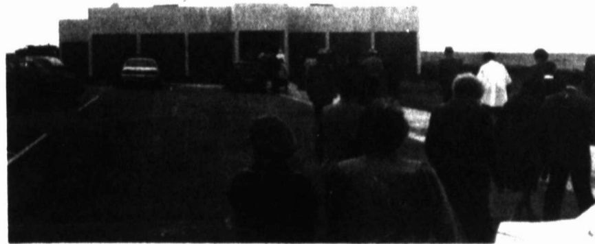
THE NEW COURSON RFO BUILDING was dedicated Sunday. A large crowd turned out for the event.
