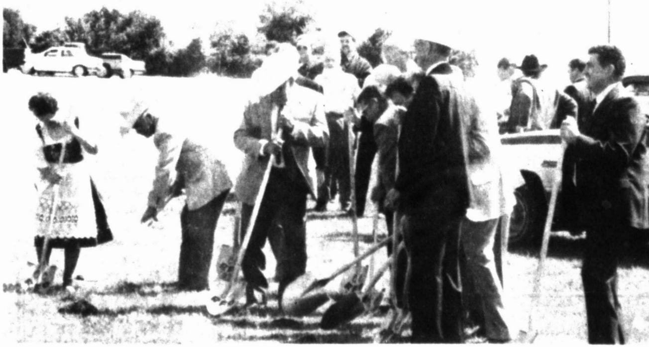
DONORS, boardmembers and guests turned sod to get the building process started.
