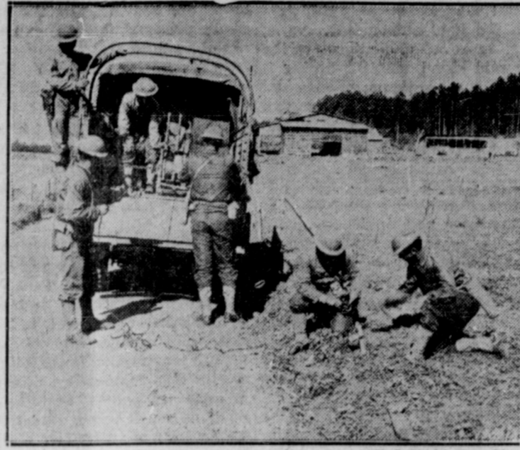
U. S. Signal Corps Photo WIRE LAYING CREW—Members of this Signal Company in southern maneuvers are changing a drum of wire and putting loading coil into line between mile-long sections. In a few minutes messages will flash between headquarters to points near the front line.
