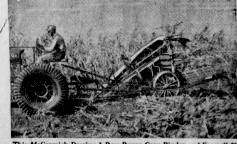
This McCormick-Deering 1-Row Power Corn Binder and Farmall 20 Tractor cut 10 to 12 acres of corn a day.
