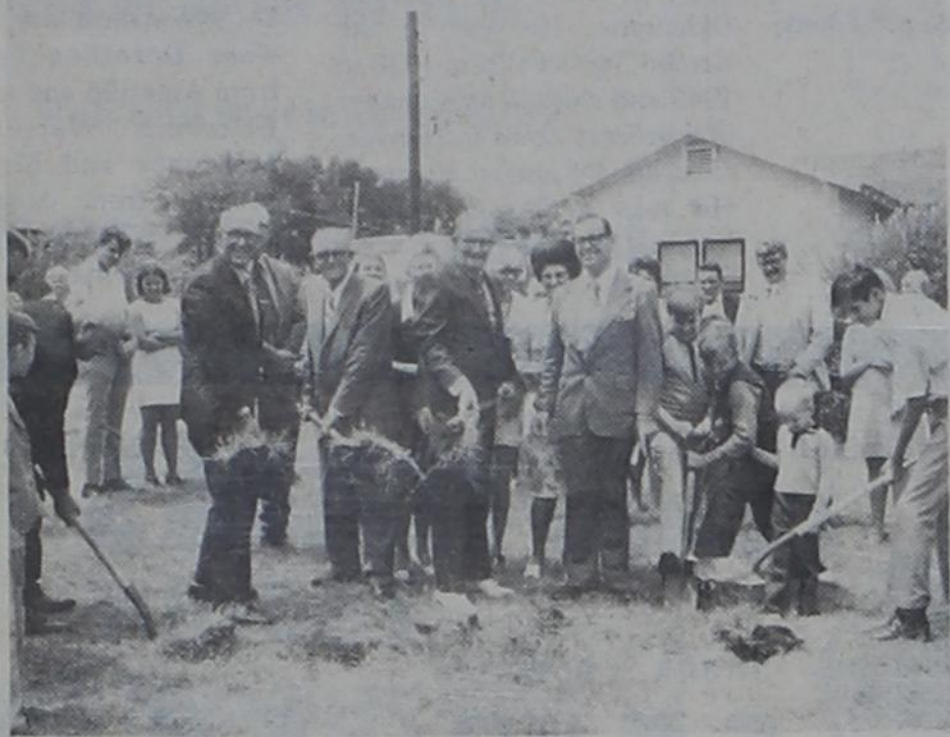
GRONDBREAKING for new auditorium.
