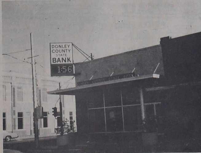
NEW SIGN at the Donley County State Bank serves as an indicator of time and temperature for local citizens and travelers.
