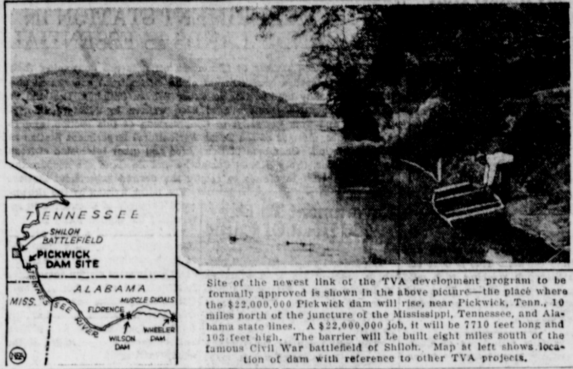
The site of the newest link of the TVA development program to be formally approved is shown in the above picture—the place where the $22,000,000 Pickwick dam will rise, near Pickwick, Tenn., 10 miles north of the juncture of the Mississippi, Tennessee, and Alabama state lines. A $22,000,000 job, it will be 7710 feet long and 103 feet high. The barrier will be built eight miles south of the famous Civil War battlefields of Shiloh. Map at left shows location of dam with reference to other TVA projects.
