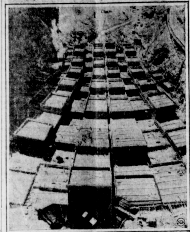
No, these aren't berry boxes piled in rows. They are sections of the foundations for Boulder Dam, the government's $165,000,000 hydroelectric project on the Colorado river. The size of the foundation works, which are built of concrete and steel, may be gauged by the small figures of men working on their surfaces.
