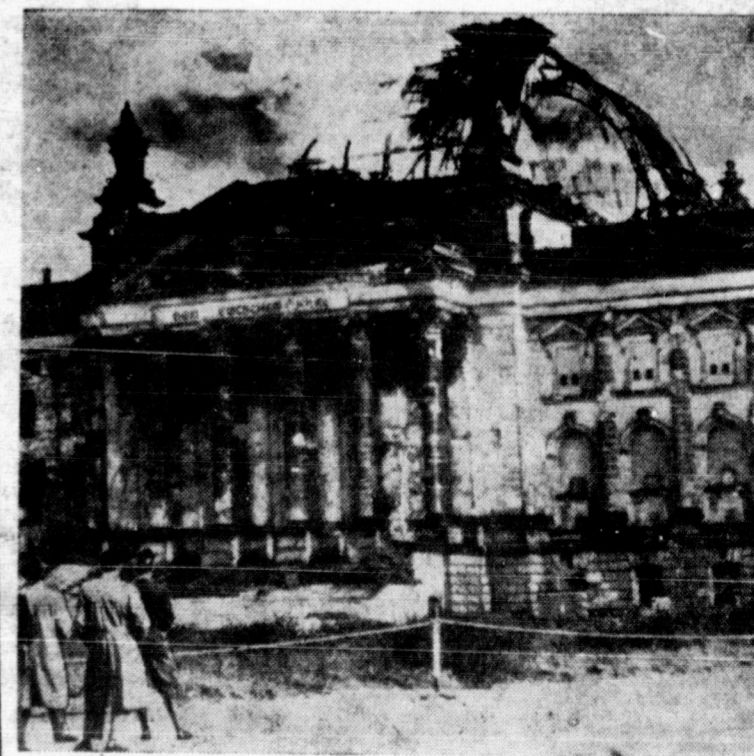
INDOMITABLE DOME . . . Berlin demolition engineers using thermite fall to topple dome of Reichstag which survived 1934 Nazi fire and World War II bombings.
