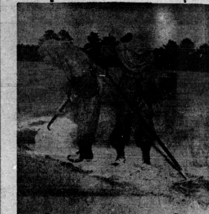
DECONTAMINATORS —Wearing fully impregnated uniforms and gas masks, two students of the Chemical, Biological and Radiological School at Fort Bragg, N.C., work a super tropical bleach into the ground. This is part of the training they receive in ridding an area of residual contamination.
