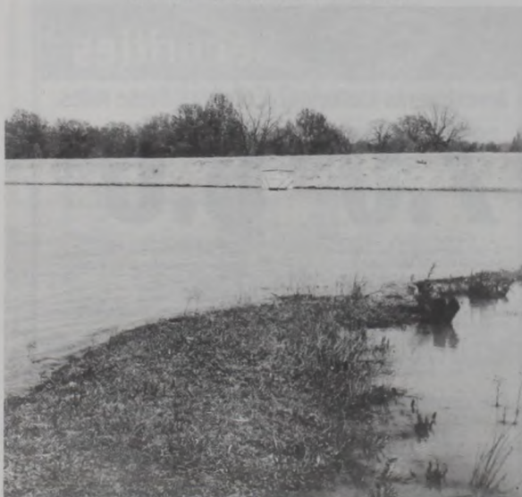
Stockwater pond with principal spillway on the Clayton Brooks farm - 1968
