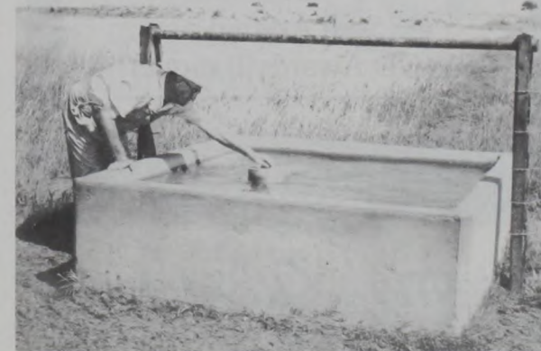
Tony Walterscheid adjusting float on completed water trough - 1968
