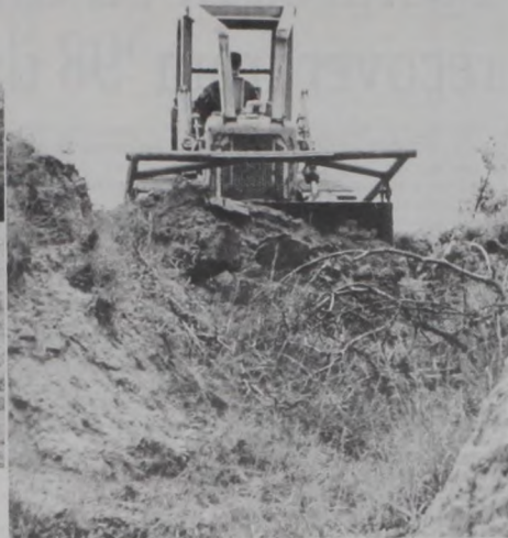
Bill Harris, last years Zone III conservation winner continues the practice on his farm north of Saint Jo. The diversion and grade stabilization structure should help control erosion and run off so the damaged can be dozed and repaired.
