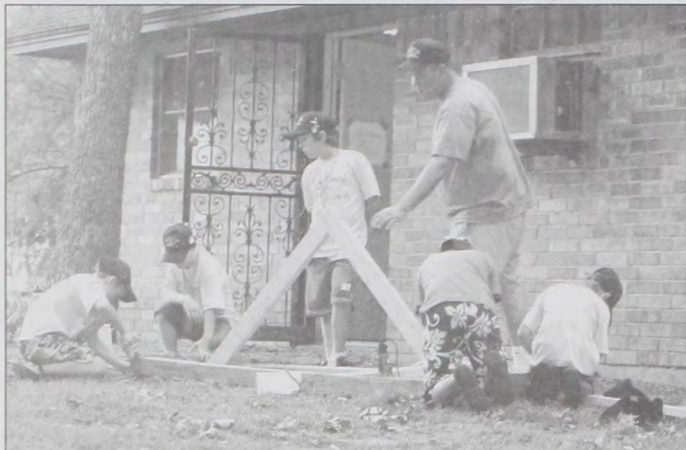
Zane Kemp, Daniel Hess, Devon Hacker, leader Ray Bell, Kyle Klement, and Justin Ashley work on the construction of a catapult.
