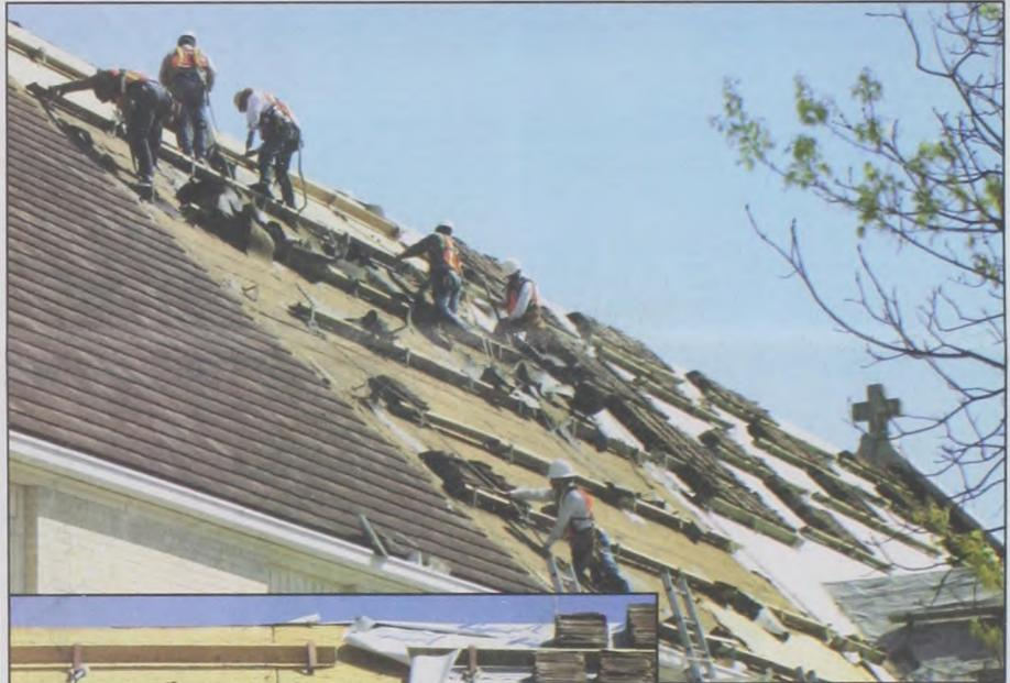
Repair work continues on Sacred Heart Church as workers removed the old roofing tile and are replacing the underlayment (as pictured) and damaged wood on the roof. The Church is also being tuck-pointed, the cutting out of old mortar and replacing it with new.
