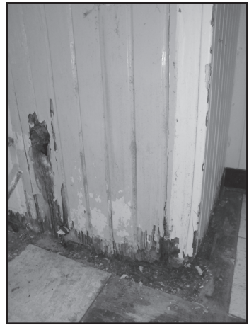
The old practice gym (built in 1949) has safety issues: the floor has sunk over six inches in some areas; there is termite and water damage. The practice gym is necessary to allow all ten school teams time to practice.
