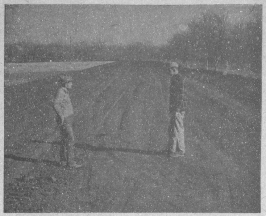
JOHNNY BAYER and Emmitt Yoder inspect a shaped waterway on the Bayer farm near Muenster. The wide flat waterway has been sodded to bermudagrass and will act as a safe outlet for a diversion terrace that will protect the bottomland field from outside hill water.
