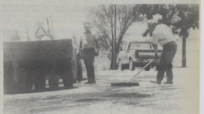
MICHAEL K. LEWIS and Lisa Hoedebeck sweep dirt and loose gravel from pot holes to ready them for a mopping with hot oil. After the mopping, Kevin Bell, Carmen Dougherty and David Dittfurth fill the holes with asphalt. Joe Fenton uses a lute to smooth the filled holes, and Wayne Tate waits to roll the filled hole down pat.
