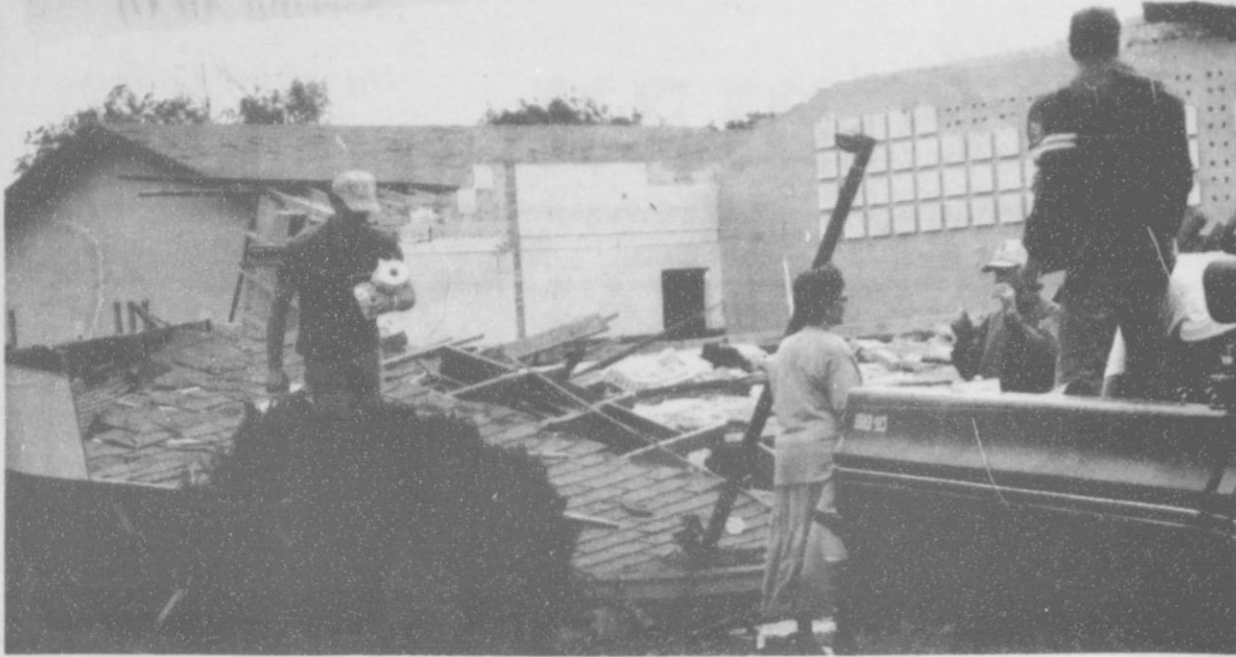
John Scott (left) and volunteers work to salvage what they can from the Church of Christ building destroyed by a tornado Thursday night.
