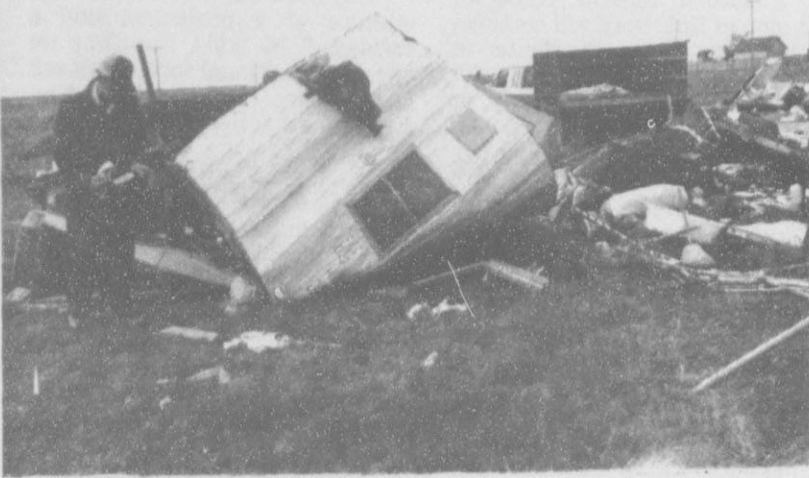
Spearman resident returns to the rubble of his trailer to dig out clothes to wear. This trailer was one of four destroyed on 7th Street.
