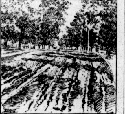
ROAD READY FOR OILING.
