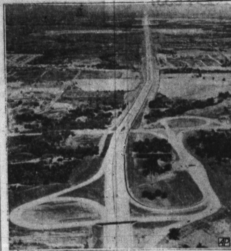
DALLAS-FORT WORTH TURNPIKE —This airview of the $58,000,000 Dallas-Fort Worth Turnpike, six-lane, divided super-highway linking the heart of Dallas with the heart of Fort Worth, a distance of 29.6 miles; is shown stretching west from a point just west of Grand Prairie. (AP Photo)
