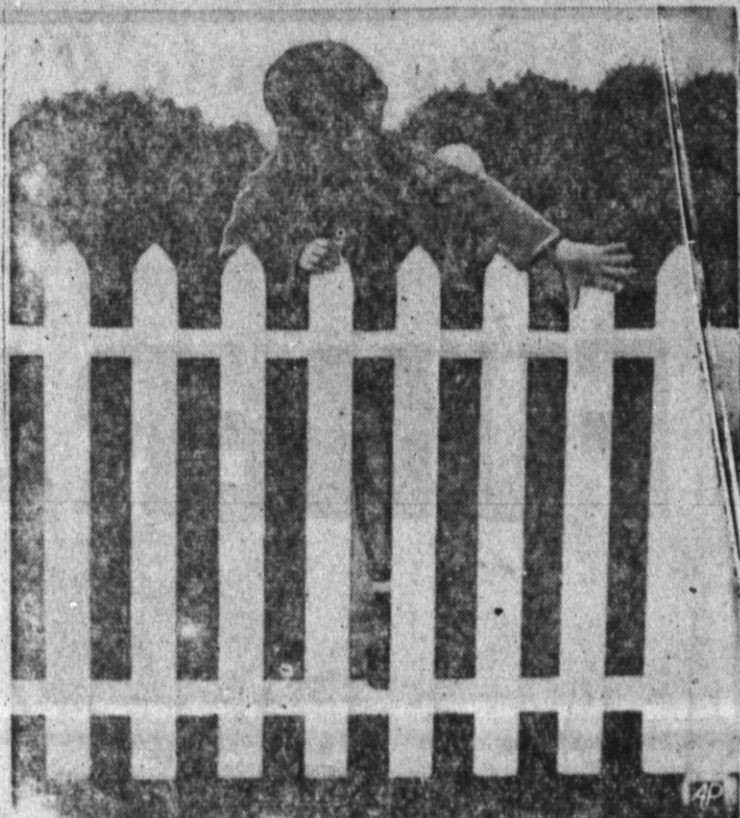
DECORATIVE DANGER—This picket fence is pretty, but it's a hazard. One slip in the operation above and a boy might be seriously hurt. Such fences can be made safer by sawing off the pointed tips.
