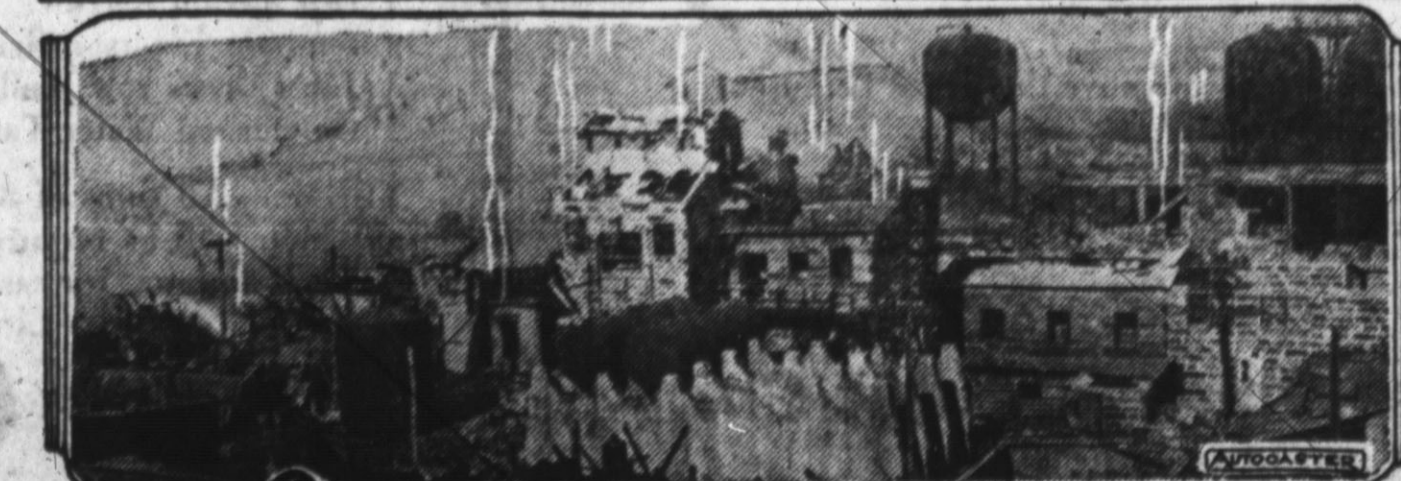
Scene of the terrible blast in a nitrate plant at Nixon, N. J., where war materials were being salvaged to make fertilizer. The shock of the explosion was felt in New York City and for a distance of 20 miles.
