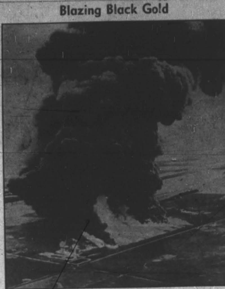
Destroying oil at the rate of $50,000 worth a day, this gusher burned and smoked for nearly four days before fire fighters succeeded in quenching the blaze. The fire threatened the $300,000,000 Ludec oil fields near Edmonton, Canada. Firemen extinguished the flames by forcing water down nearby relief wells.
