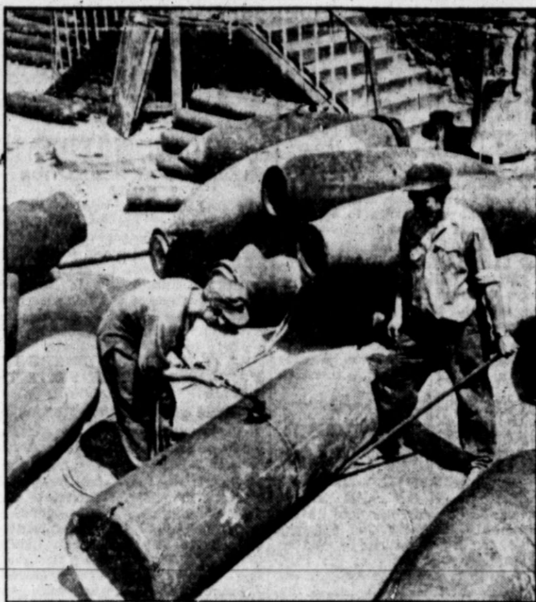
LEFT OVER FROM THE BLITZ —Workers in Berlin use an acetylene torch to carve up a two-and-a-half-ton blockbuster for scrap. Originally destined for England via the Luftwaffe, the bombs are among hundreds of tons of scrap iron and steel being shipped daily to England by a more peaceful water route.
