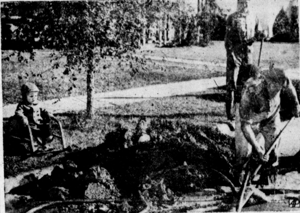
SIDEWALK SUPERINTENDENT, JUNIOR GRADE —Little Tommy Peurifoy, 2 years old, got on early start on the popular pastime of kibitzing when a water main broke in front of his Dallas home. Workmen had not been on the job long when the young son of Mr. and Mrs. T. J. Peurifoy placed his rocking chair where he could comfortably observe and supervise the project. (AP Photo)
