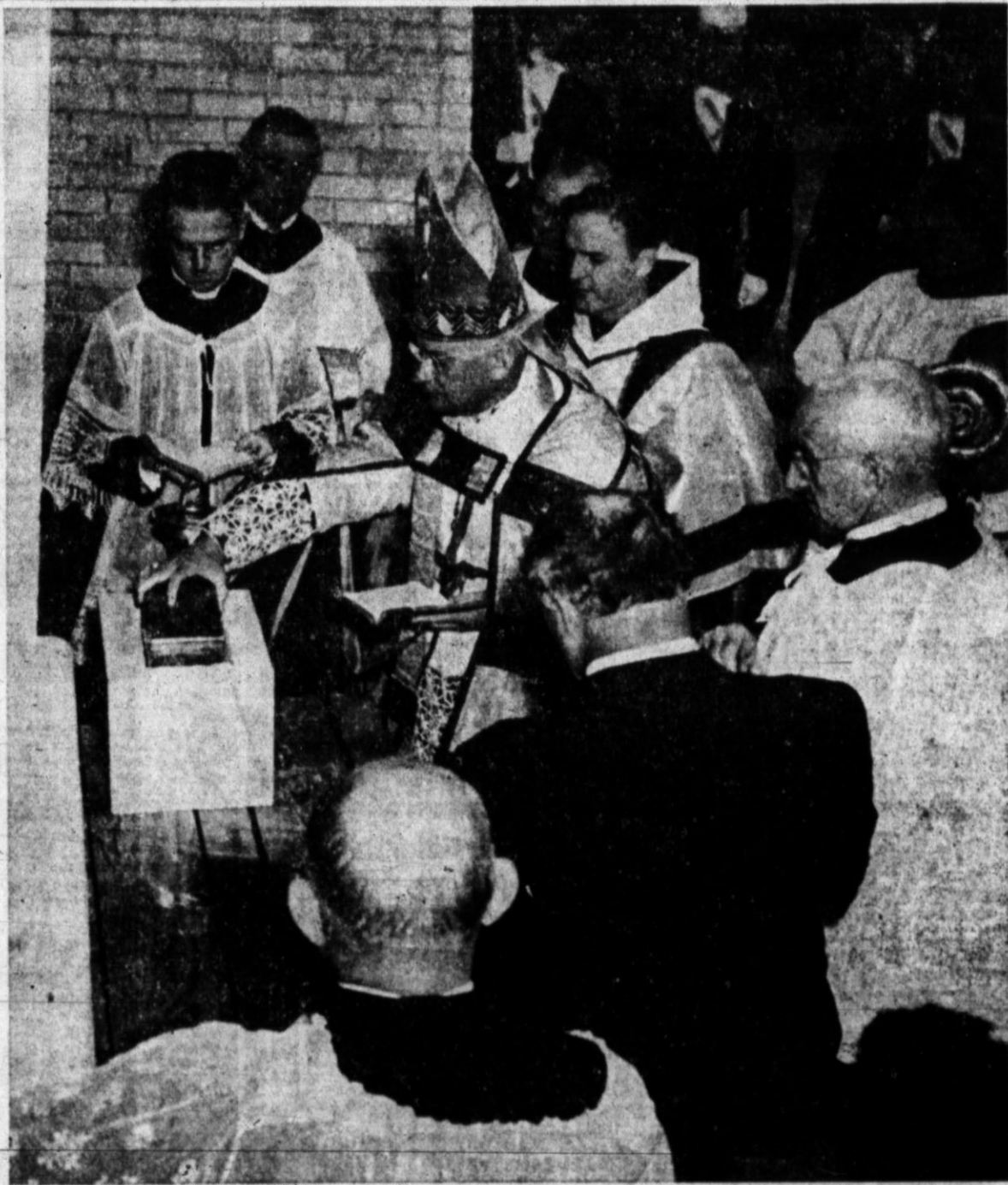
HISTORICAL DOCUMENTS being placed in the cornerstone of the St. Anthony's Catholic church are deposited in the above picture by Bishop Laurence FitzSimon, bishop of the Amarillo diocese.
