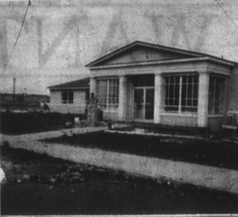
NEW ENTRANCE — Visitors to King Manor "open campus" Sept. 4 will find a much larger lobby than the original building boasted. This is the entrance to the new part, nearing completion. A portion of the hospital is shown in left background. (Brand Staff Photo)
