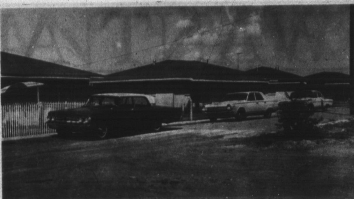
NEW DUPLEXES — King's Manor and West-gate have several new buildings, among them new employees' duplexes. All were shown at last Thursday's "open campus" at Kings Manor. (Brand Staff Photo)
