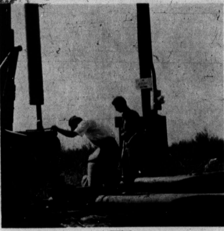
Pulling pipe preparatory to changing pump. Turkish engineers inspect.
