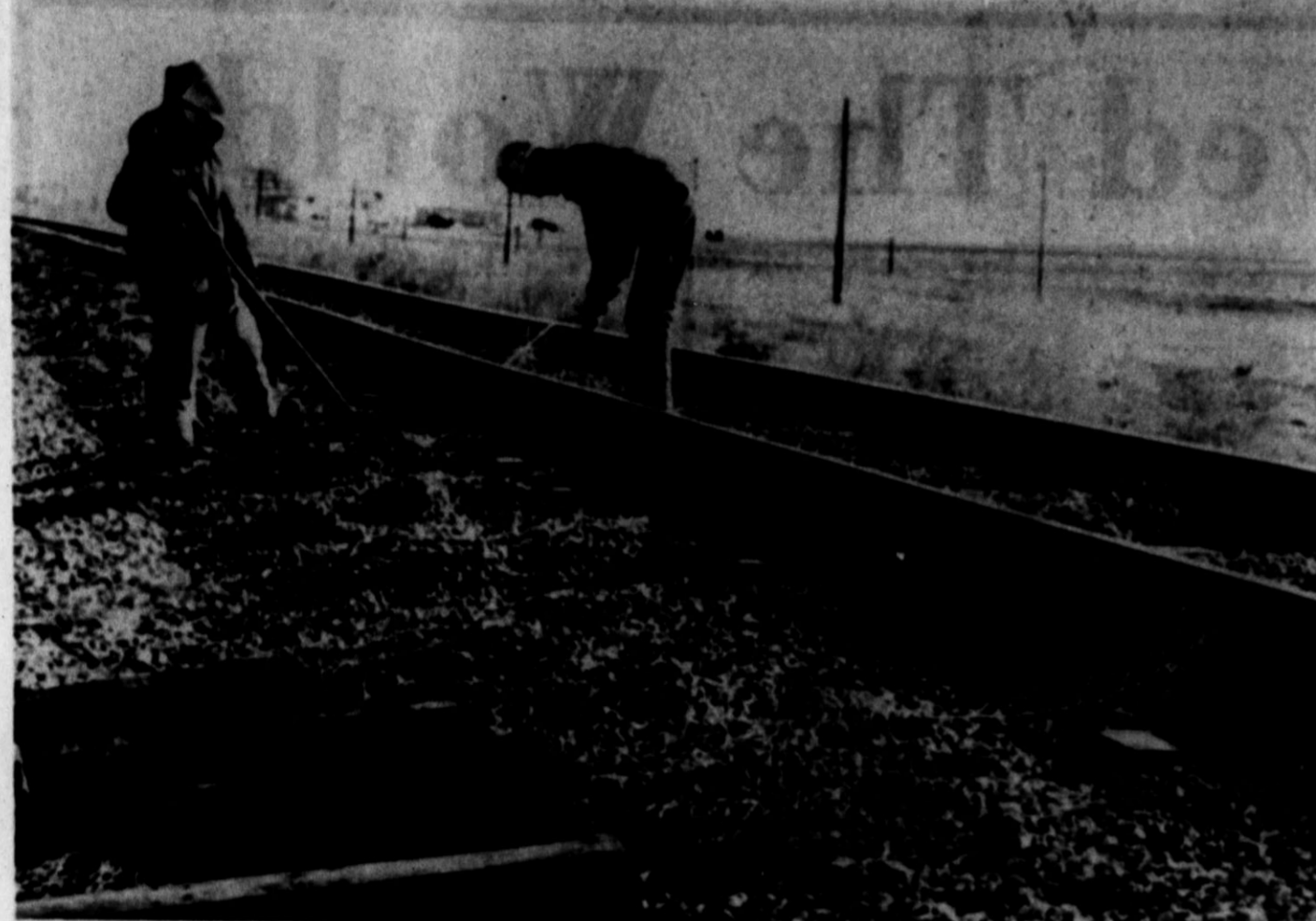
Working on the Railroad
