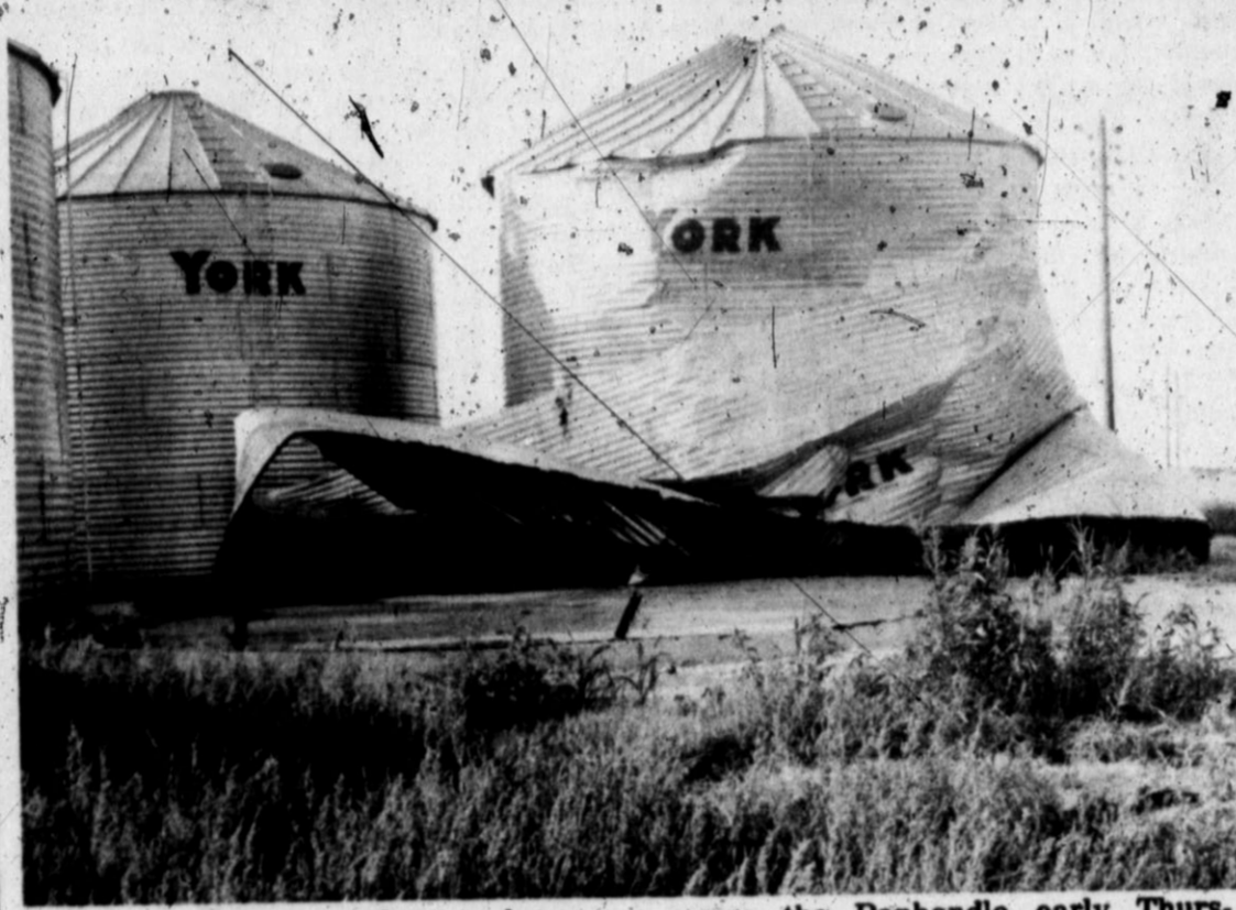
WIND DAMAGE — One tank was destroyed and another damaged at Miller Seed Company when winds clocked at 60 miles per hour swept across the Panhandle early Thursday morning. Damage at Miller Seed was estimated to be at least $7,000. — Staff Photo
