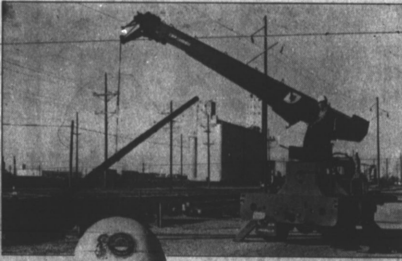
"Johnnie, what are poles costing these days?"
