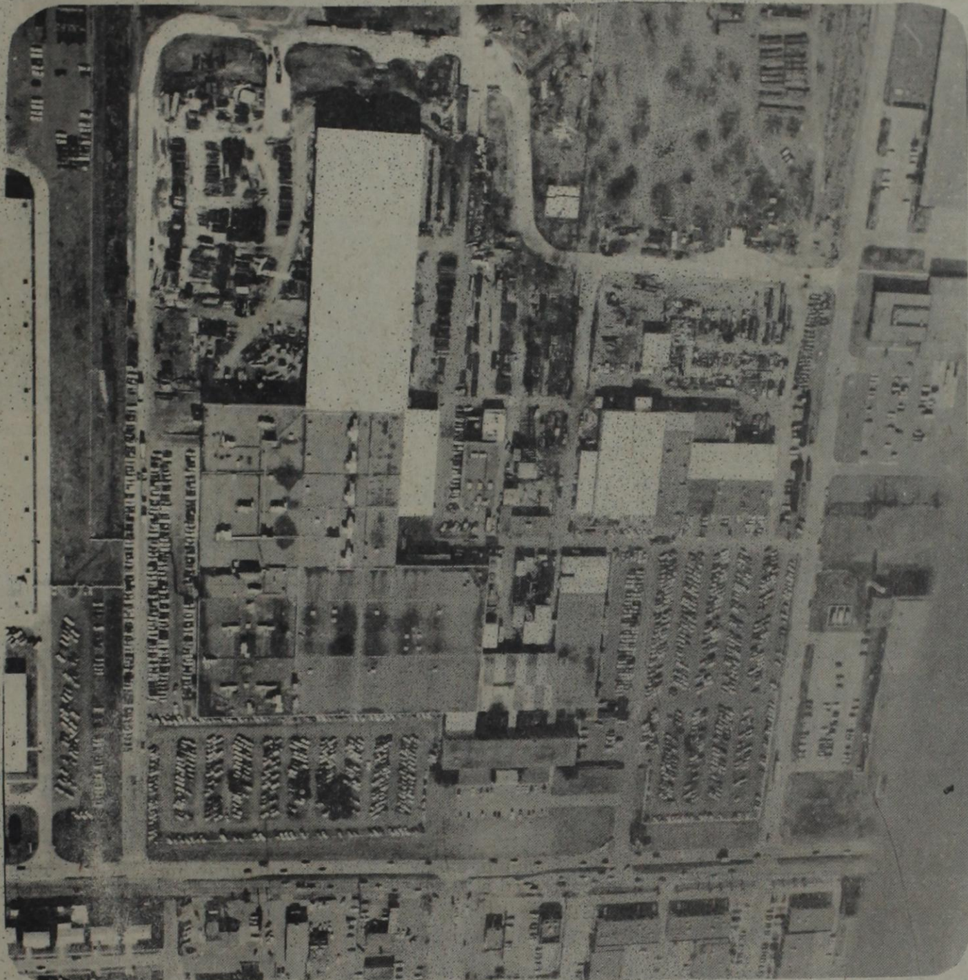
67 acres, over 30 acres under roof-expanding everyday, Dallas Facilities
