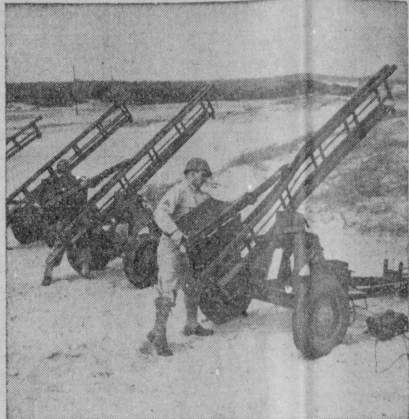
ARMY'S NEW ROCKET GUNS —When the enemy perfects jet-propelled planes, Yank anti-aircraft gunners will be ready. Artillerymen at Camp Davis, N. C., Holly Shelter Range, are using jet-propelled rockets that rise from specially designed carriages at velocity of 450 miles per hour as targets to stimulate diving enemy planes. Using .50 calibre machine guns and 20 and 40 mm. weapons to track fast-moving, 50-inch targets that describe a parabola and have maximum horizontal range of 2,200 yards, develops bulls-eye accuracy. Photo above shows how jet-propelled rockets are loaded onto launching carriages. One fin fits into narrow groove between railings that form nose of carriage.
