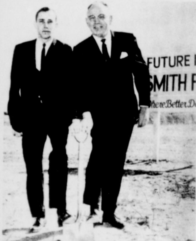
TEAMWORK — Bill Smith and son Steve teamed up on the shovel to break ground for the new Smith Ford, Inc. building here
