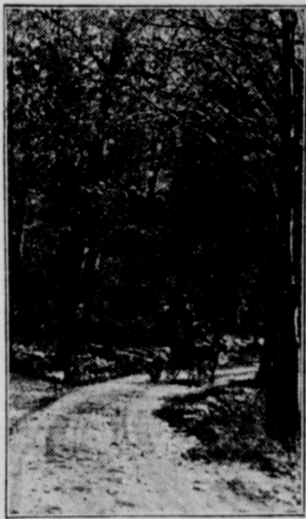
Improved Road in the Woods.
